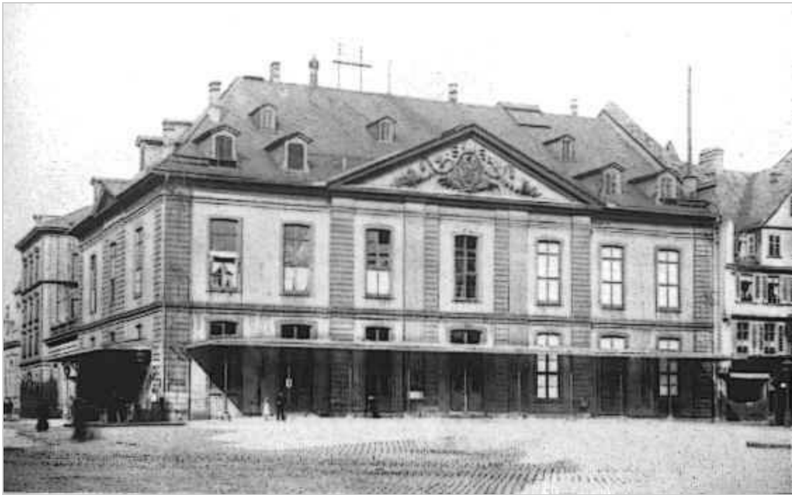
The Comödienhaus in Frankfurt in 1902, shortly before it was torn down
